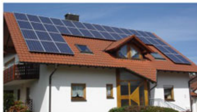
Off-grid Home Solar System
