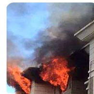
Life and property will be gone if home occur fire caused by gas leakage
