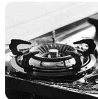
The gas stove going out unexpectedly cause gas leakage
