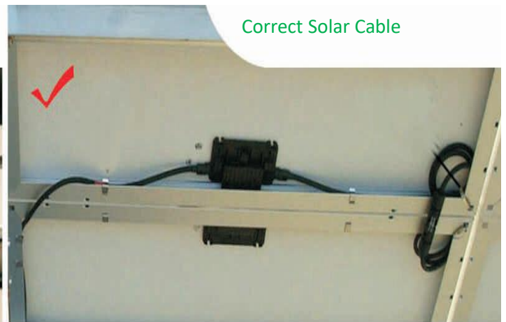
Correct Solar Cable
