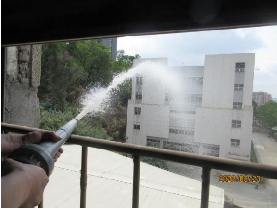
Fire hydrant testing
