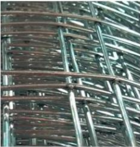
Galvanized before welding
