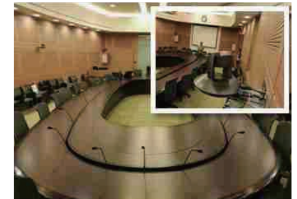
HD PTZ Cameras Installed at Israel Parliament
