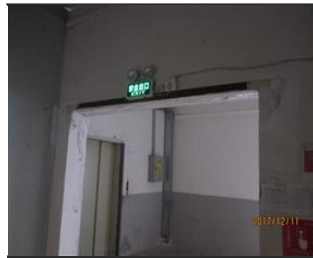
Photo of fire safety equipment Safety exit with emergency light and exit sign.JPG
