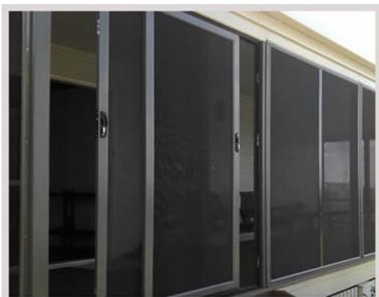
High tensile 316 marine grade stainless steel mesh used for door screen
